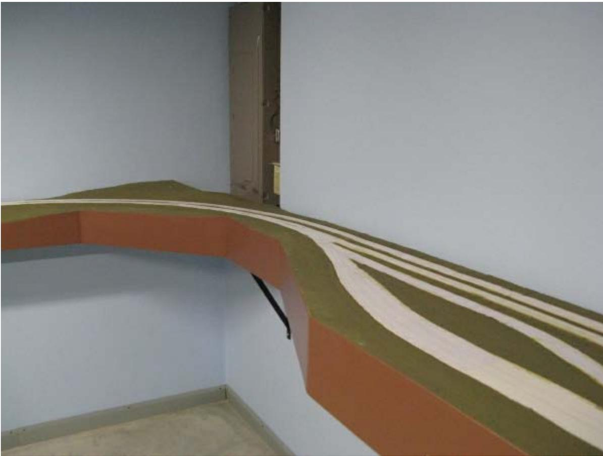
**Left:** The fascia is now painted and the base color has been painted on the scenery plaster. I use interior latex semi-gloss paint on the fascia board. For the scenery base coat, I use interior latex flat paint. I keep the paint off the paper track templates, which were glued in place when I installed the roadbed. This area is now ready for track!
