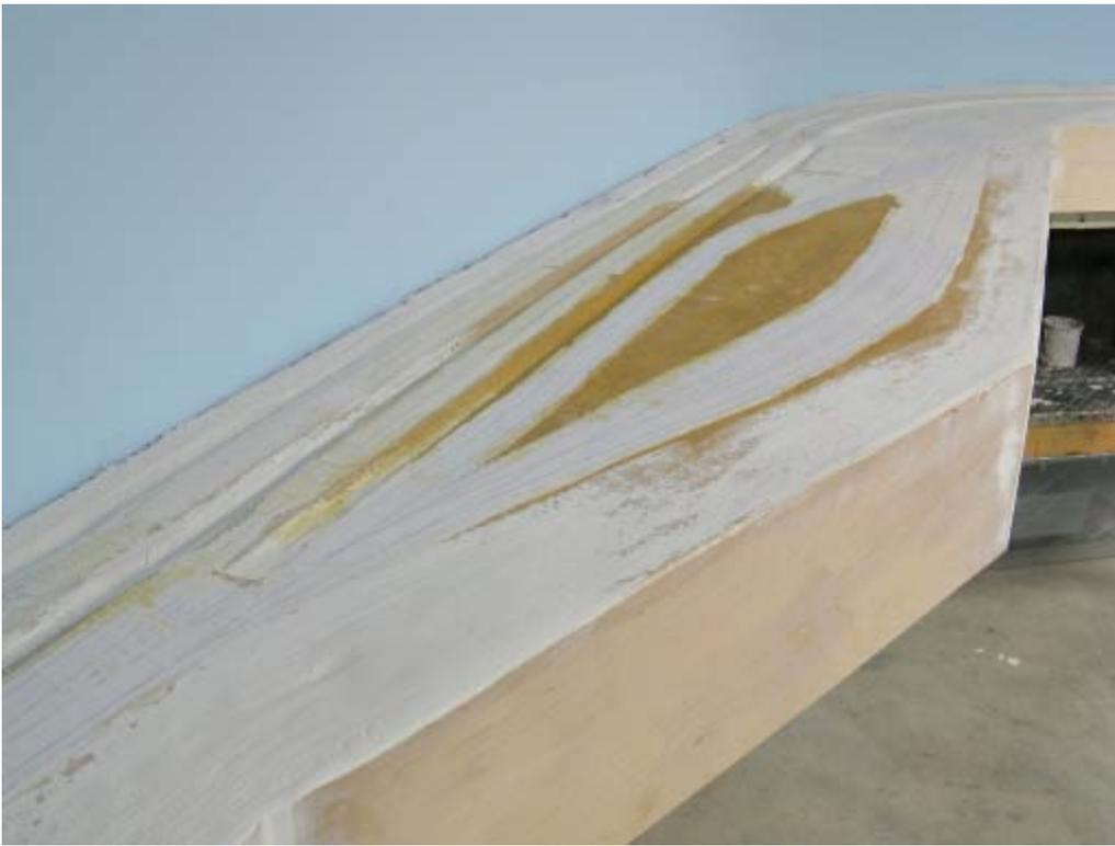
**Left:** In this picture, the fascia board is installed and the plaster coat has been added over the pink foam board. The fascia is made from ¼" plywood. When I'm working on the scenery plaster, I use some of the plaster to fill any nail holes or blemishes in the plywood.
