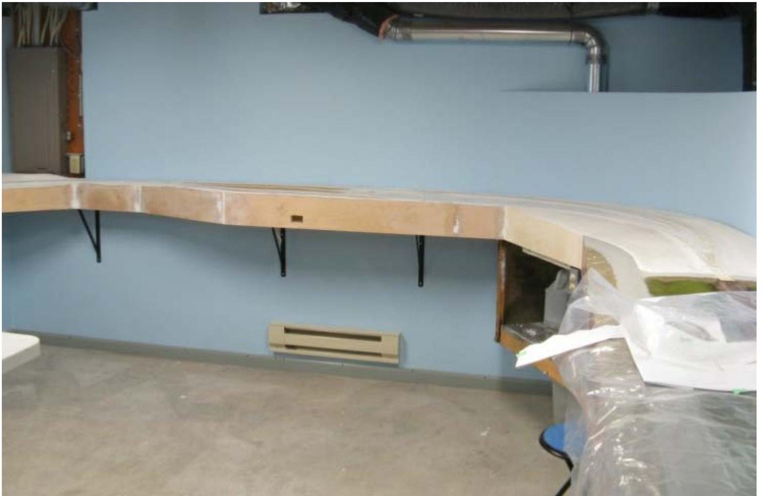
**Above:** This is a view of the overall area of this season's work. When working with plaster and paint, I cover the nearby finished areas with plastic sheeting. At this point, the plaster used on the fascia has been sanded smooth.
