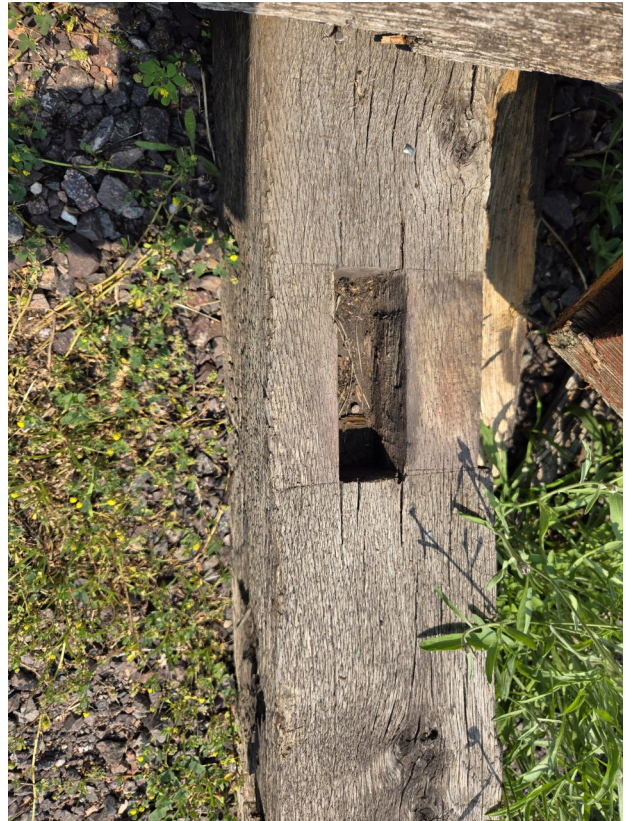
Portion of the side sill from rock car #36 showing the original layout lines for a mortise for one of the upright side posts. These were marked out using a knife and/or a carpenter's marking gauge, then opened with an auger drill and chisels.
