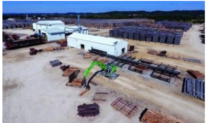
The Stella Jones Railroad Tie Treating facility.
