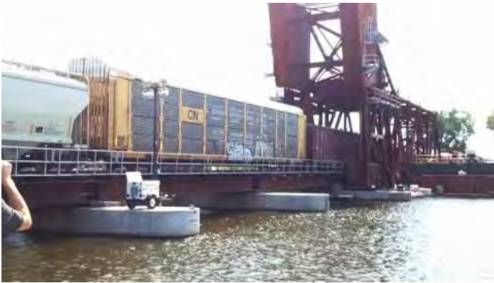
Below, a train goes through the newly completed bridge.
